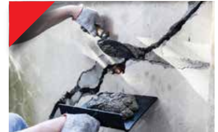
Cracks Repair
