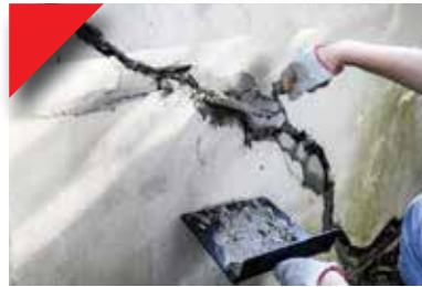
Cracks Repair
