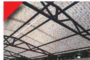
Precoated Sheet Fitting
