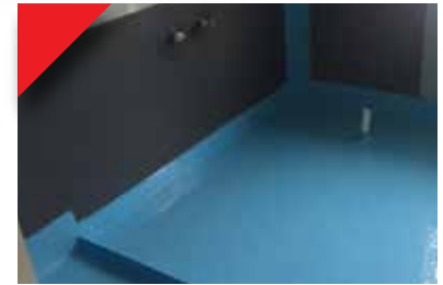
Bathroom Waterproofing
